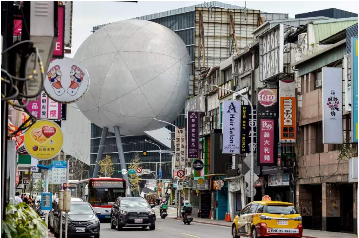
Taipei Performing Arts Centre © Chris Stowers
