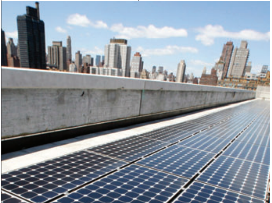
THE 50KW ROOF-INTEGRATED PHOTOVOLTAIC ARRAY (ABOVE) IS THE LARGEST IN MANHATTAN, PRODUCING ENOUGH ELECTRICITY TO POWER ALL OF THE OCTAGON’S COMMON AREAS, CORRIDORS, ELEVATORS AND LOBBY. THE COMMUNITY’S MYRIAD GREEN FEATURES INCLUDE ROOFTOP HEAT RECOVERY UNITS, NET ELECTRICAL METERING, OCCUPANCY SENSORS AND A SWIMMING POOL THAT IS CONNECTED TO THE BUILDING’S WATER LOOP TO IMPROVE EFFICIENCY OF SUMMERTIME COOLING.
